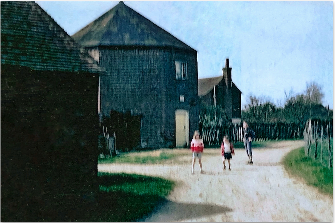
Old Mill House in 1968.
